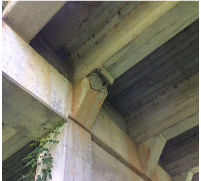
PHOTO 2 Description Repair delaminated under Girder # 2. Bent # 5.
