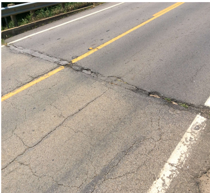
PHOTO 4 Description Expansion joint over Bent # 1.
