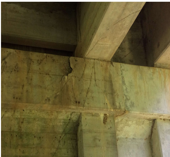
PHOTO 4 Description Delaminated area in Span # 8 side of Bent # 9 cap under Girder # 4.
