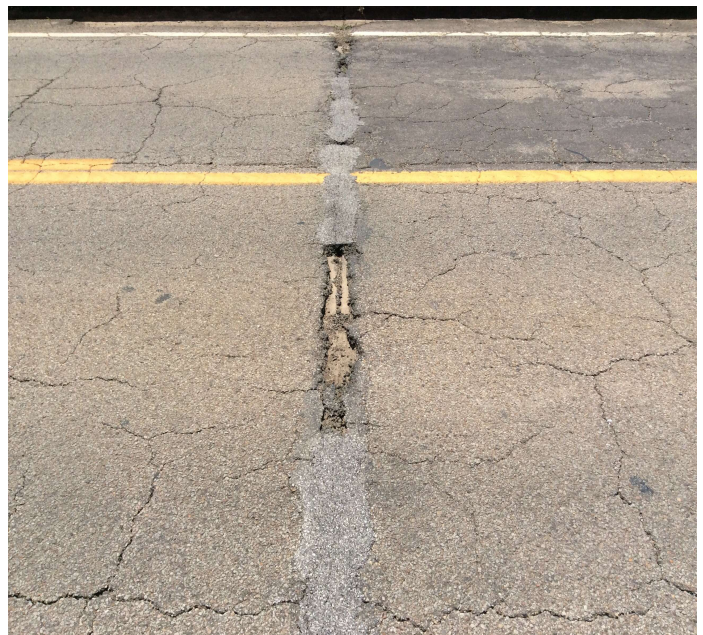
PHOTO 2 Description Expansion joint over Bent # 3.
