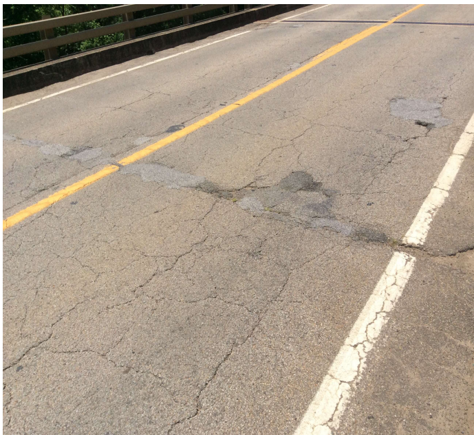
PHOTO 3 Description Expansion joint over Bent # 7.
