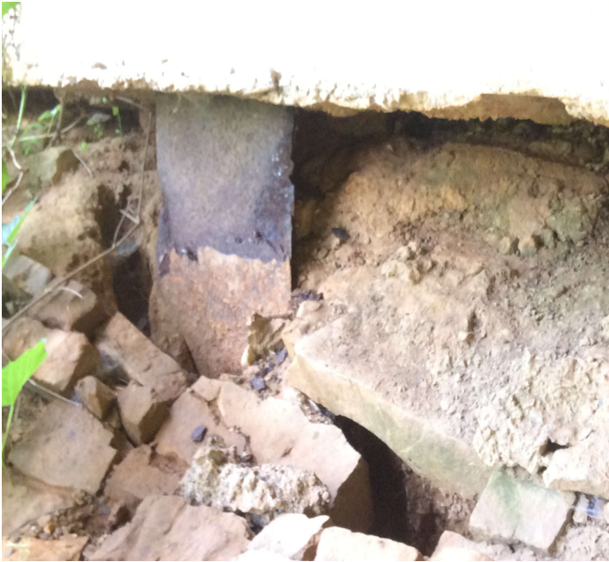
PHOTO 1 Description Bent # 11. Left piling . Knife edge section loss.
