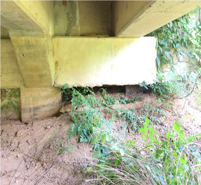
PHOTO 3 Description Bent # 1. Left side. Exposed Piling.
