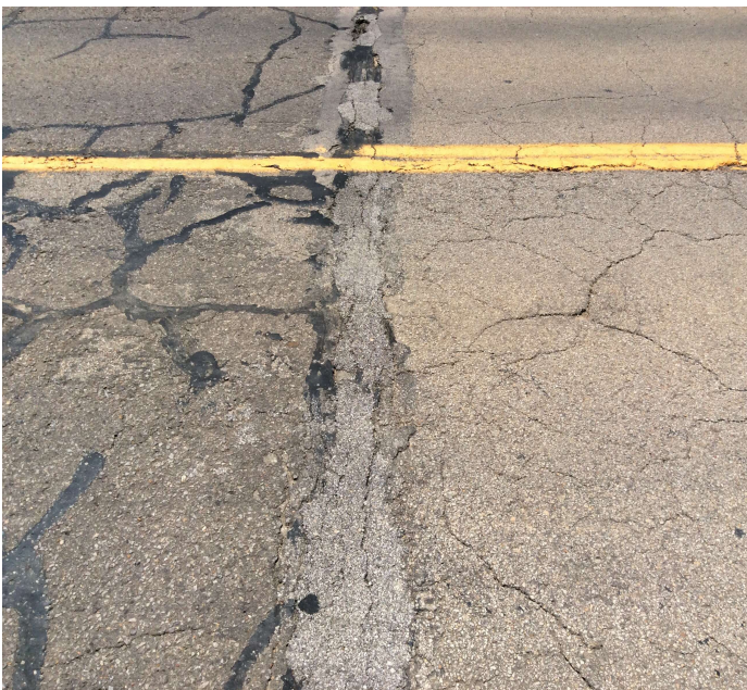
PHOTO 1 Description Expansion joint over Bent # 11. East abutment.
